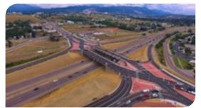
Constructing the I-25/Fillmore Diverging Diamond Interchange while maintaining traffic flow presented project phasing challenges. To deliver the project on time. SEMA proposed adjustments to the original 16-phased sequence plan, including implementing two fast-track weekend closures when traffic was lighter. that cut approximately two months from the schedule.
